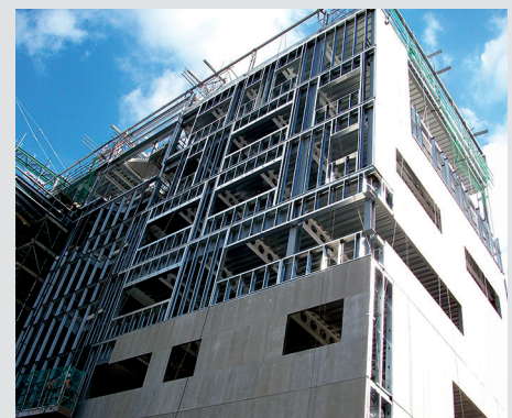
Light steel sections in an external wall application
