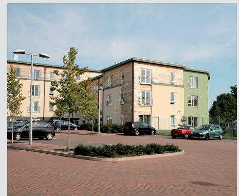
Light steel extra care housing scheme
