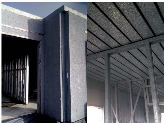
Figure 4 Light steel frame structure after 5 years exposure (Image courtesy of Fusion and Evolusion)
